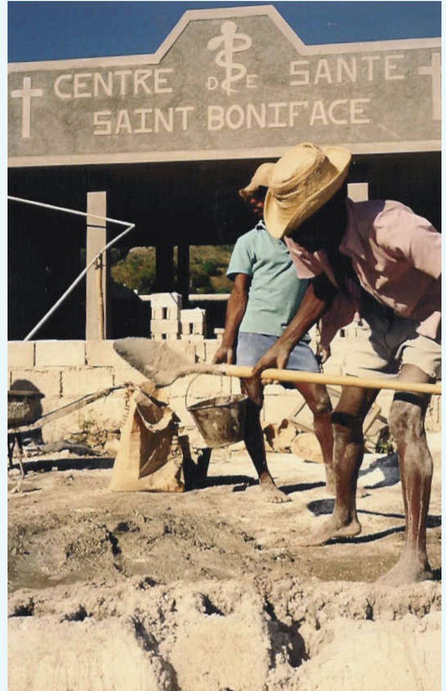
Constructing the first Saint Boniface Health Center
